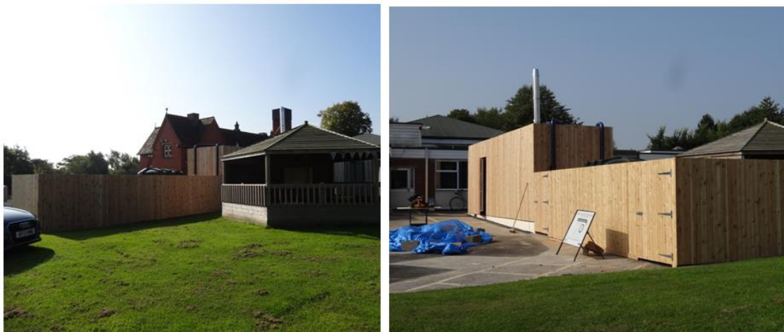
Figure 1: Yelvertoft School: view of the biomass boiler cabin and annexed oil tank enclosure from the back and the front
